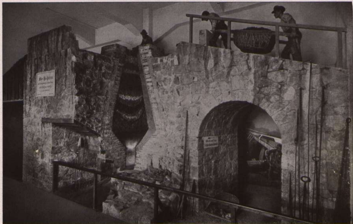
Sectioned blast furnace of 1810
