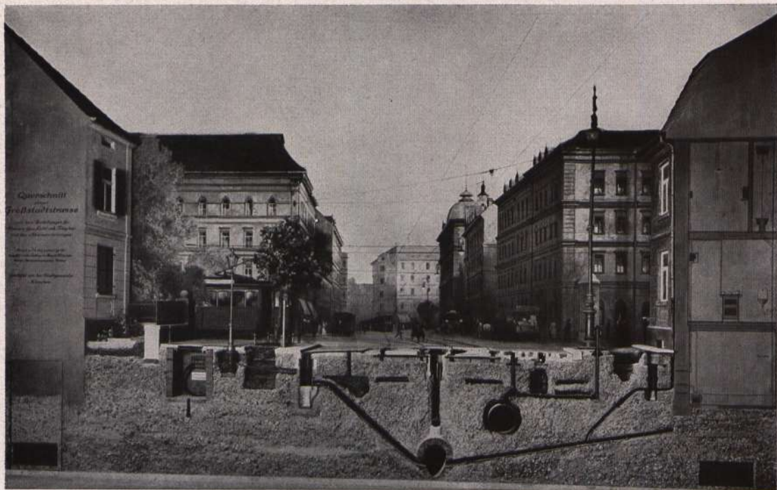
Cross-section of a modern street showing conveyance of gas, water, current, and so forth
