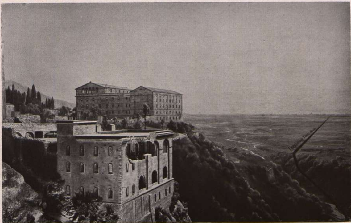
Power plant Tivoli-Rome, 1892
