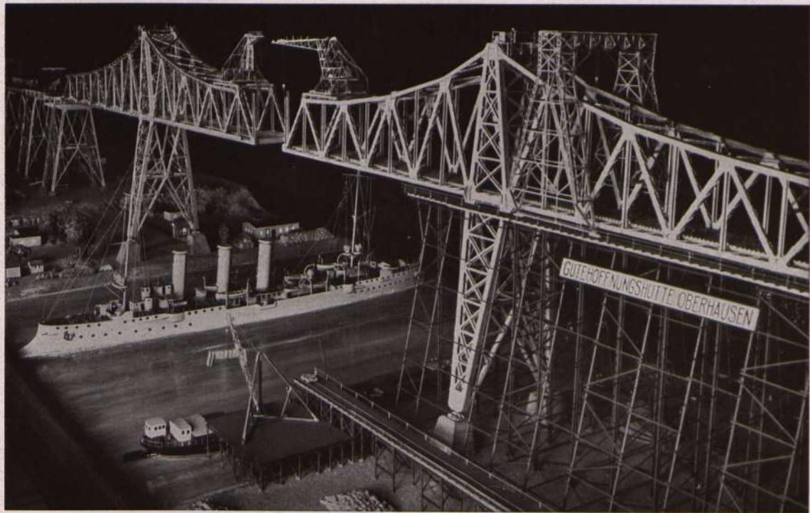
Model of an iron girder bridge in construction across the Kaiser Wilhelm Canal near Rendsburg
